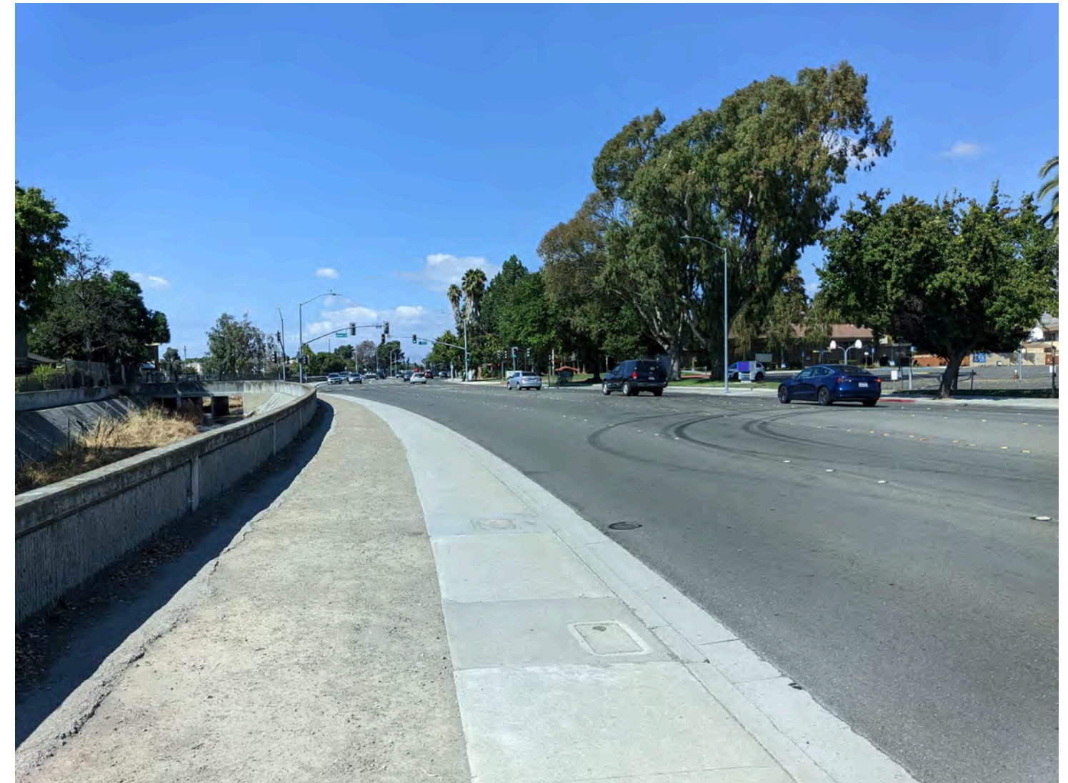
Abel St, Looking North
