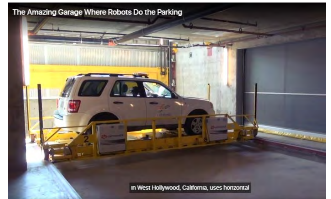
Automated parking garage.
