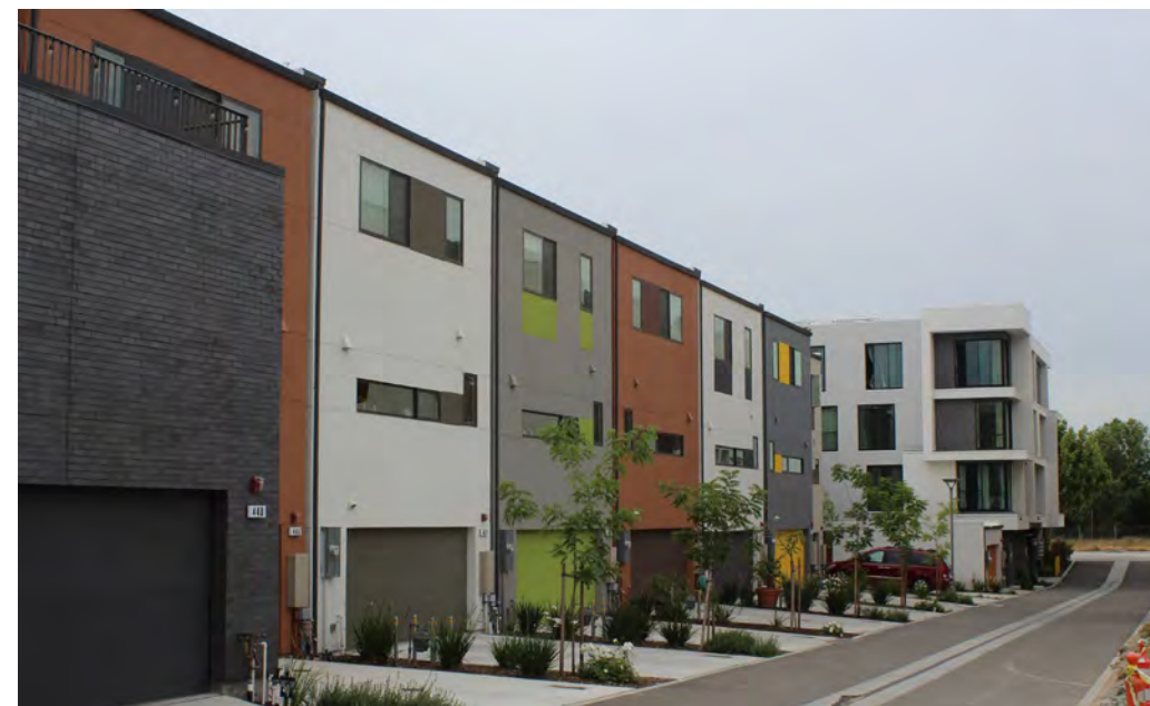
Townhomes with tuck-under parking and apron.
