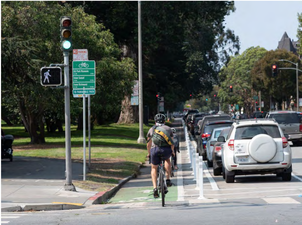
Parking Protected Bike Lane – San Francisco
