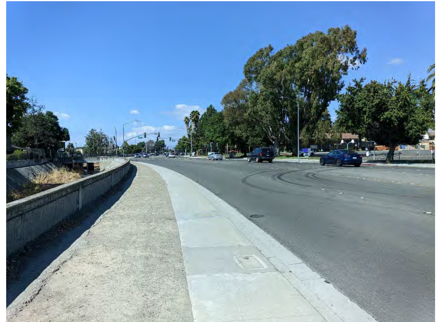
Abel St, Looking North
